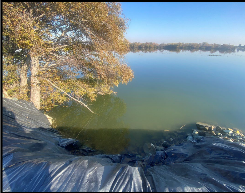
Station 256+40 – 257+00. Facing north. Dated 12-13-2023
