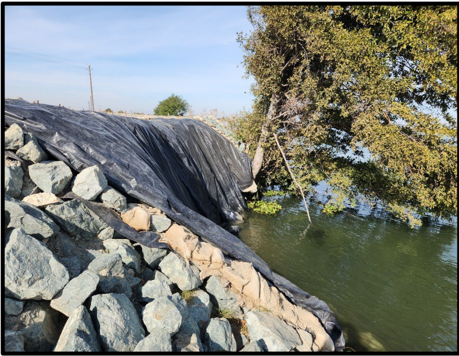
Station 256+40 – 257+00. Facing west. Dated 11-13-2023
