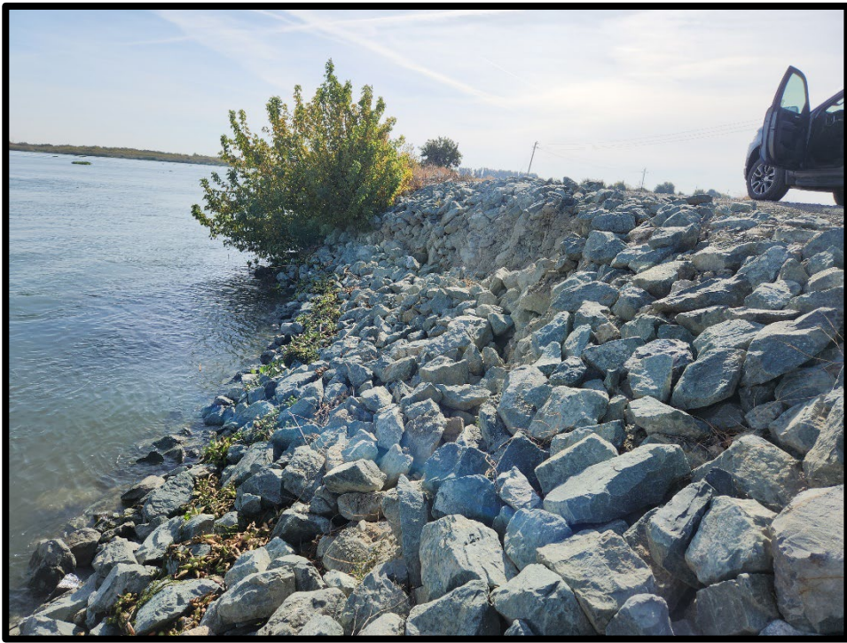
Station 255+50 – 256+20. Facing east. Dated 11-13-2023
